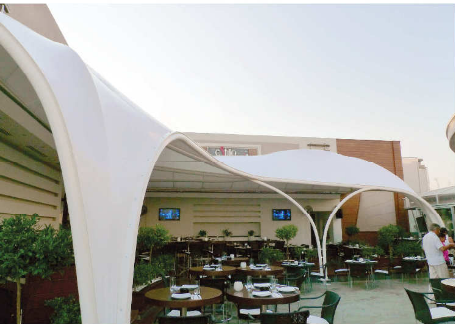
Cipro - project: Kukan architects
